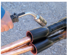
Heat shrink cable joints/splices
